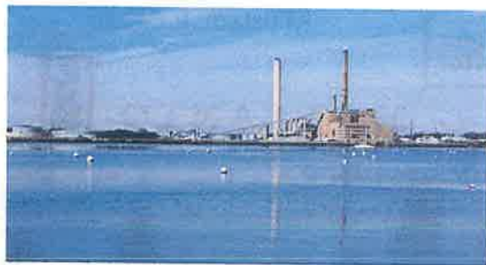
Old Salem Harbor Station (2014)
